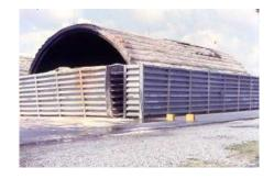
One New Hardened Shelter. Air revetments are good for protecting aircraft but the ultimate upgrade is the hardened shelter. This unit can protect your valuable aircraft and ground crew from attack, leaving you ready for a counter strike. A useful insurance policy. A hardened shelter takes 3 combat engineers, 3 Excavators and 50 Defence Stores to construct
